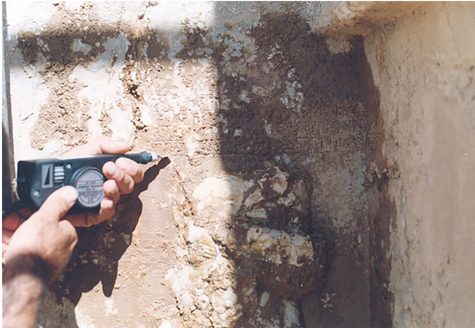
Fig. 11. Removing dirt deposits, and the lichens from DNf by Hassan Rahsaz in 2001 (© Parse-Pasargadae Research Foundation).
